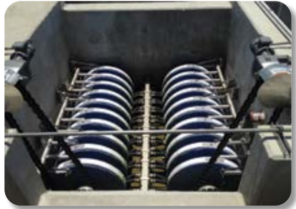
The modular design of the Aqua MiniDisk® filter retrofits neatly into existing 9 ft. (2.74 m) wide concrete traveling bridge filter basins, providing more than two times the hydraulic capacity of the original sand filters.
