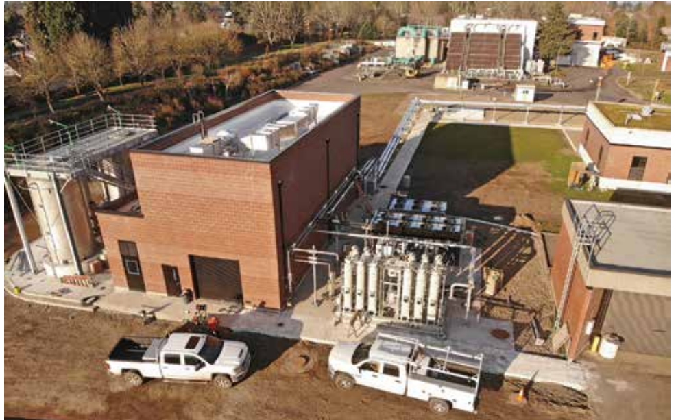
Aerial view of the Metropolitan Wastewater Management Commission plant shows equipment for purifying biogas. The Greenlane Biogas pressure swing adsorption system in the center foreground.
