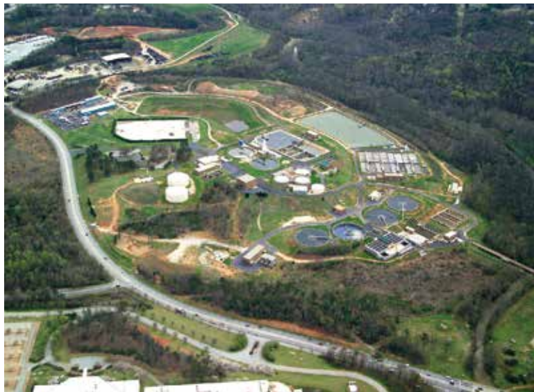
ReWa treatment facilities process more than 40 mgd in a county encompassing 795 square miles with a population of more than 500,000.
