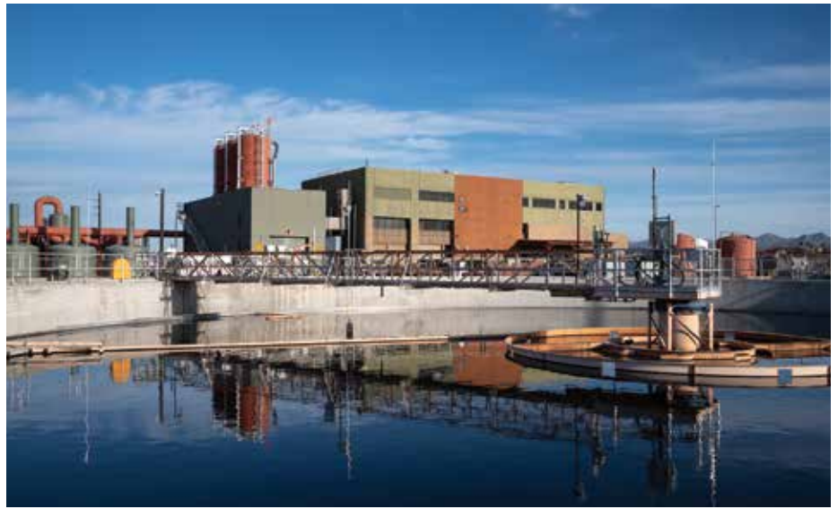
A secondary clarifier and the centrifuge facility at the Tres Rios Water Reclamation Facility in Pima County, Arizona.
