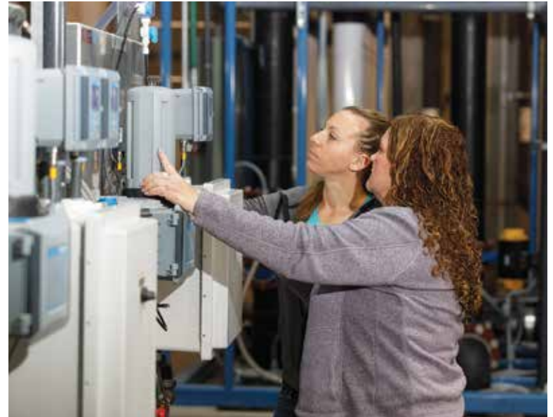
Jesse Penor (left) and Rixen calibrate a Hach turbidity meter.
