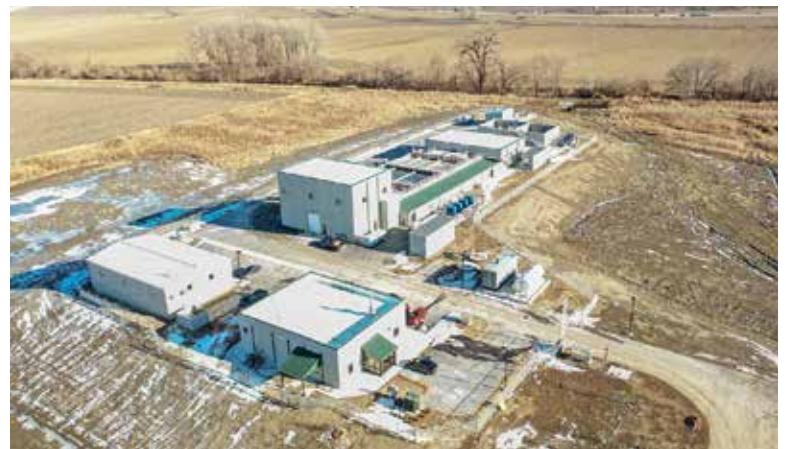
The Wolcott treatment plant rests on land that had to be filled and elevated to be above the 500-year flood plain.
