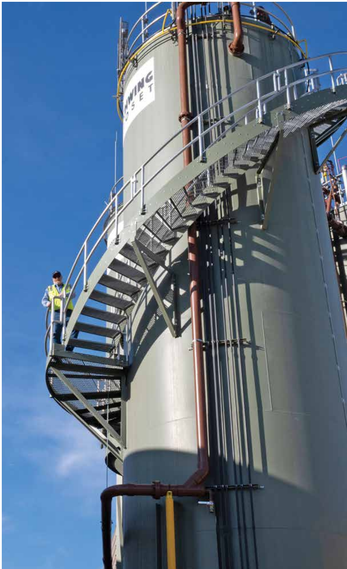
Plant manager Steven Richey with the NuReSys nutrient recovery system (Schwing Bioset).
